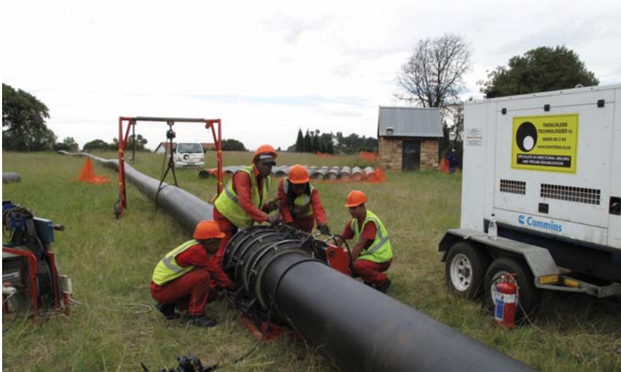
Butt-welding of 560 HDPE PE 100 PN 10 in progress
