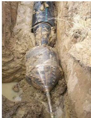
On site in Sasolburg: the 800 mm backreamer in action
