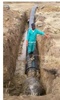
The final pull-in of the 630 mm diameter HDPE pipe
