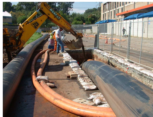
Segments of the old pipe showing damage Installation of HDPE lining in progress
