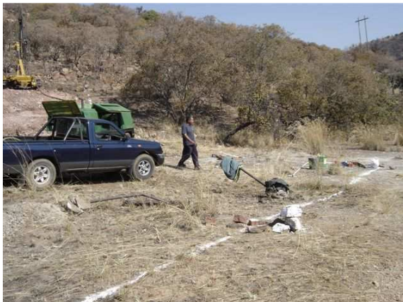
The northern approach to the tunnel after clearing. Drilling is in progress for surface blasting for the approach and the north portal
