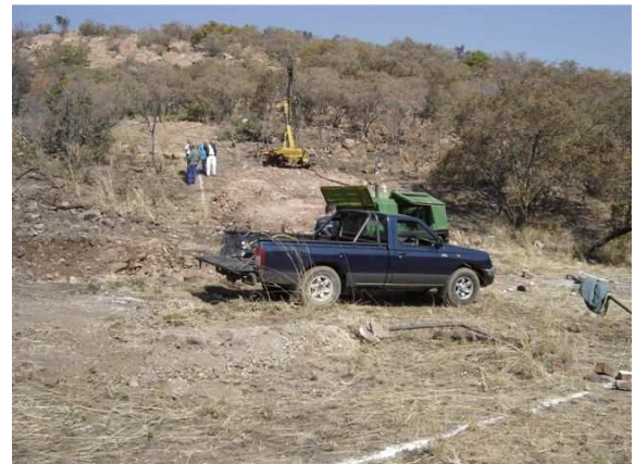
The northern approach to the tunnel after clearing. Drilling is in progress for surface blasting for the approach and the north portal
