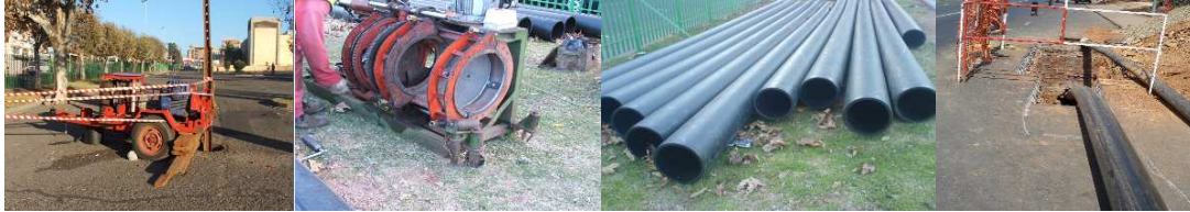
Fig 4b: Pipe Bursting (Oriental Plaza)
