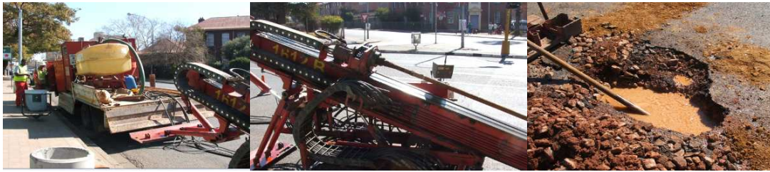
Fig 4a: Horizontal drilling equipment (Oriental Plaza)
