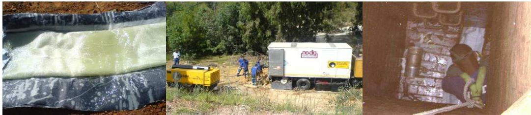
Fig 4c: Cured in place liner (Rosettenville)
