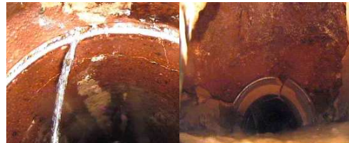
Fig. 3a: Water Infiltration
