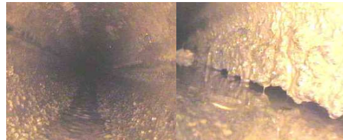
Fig. 3c: Corroded Pipe
