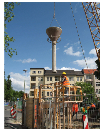
Slurry wall construction.
