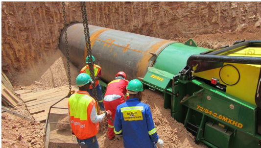
Auger boring a 1840 mm ID steel casing
