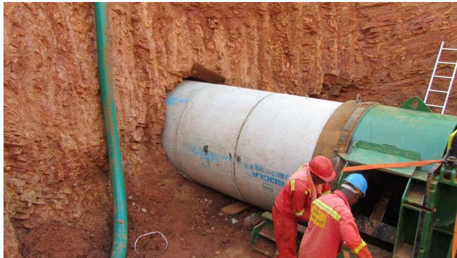
Auger boring a 1840 mm ID steel casing
