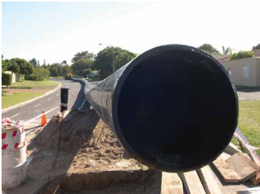
BELOW Cape Town Sliplining Pentz Drive Sewer with 630 HDPE pipe
