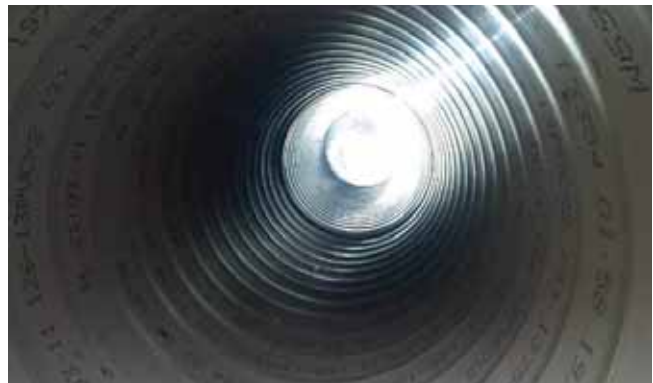
BELOW RIGHT SPR EX (Expanda) relining 600ND concrete pipes at Percy Stewart Sewage Works
